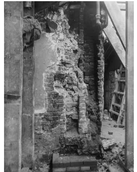
A series of photographs from 1949 recording the renovation work done to the Assembly House when various elements of the older buildings were uncovered. These included wall cores believed to be from Hobart's original Chapply Field House and the remains of a wooden, 12-light Tudor window buried behind a screed coating in the north wall of the west wing.
