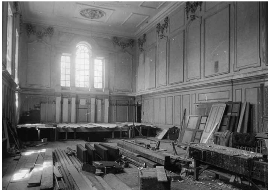
Above right: The Music Room with the gallery removed and the platform under construction, 1948/1949.
