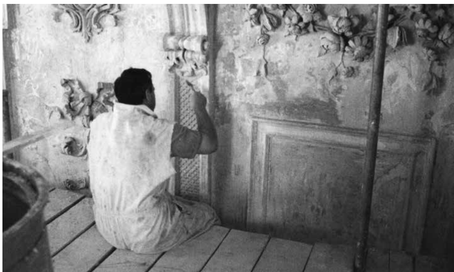
Top left: Making replacement plaster detailing and repairing sections of existing work.
