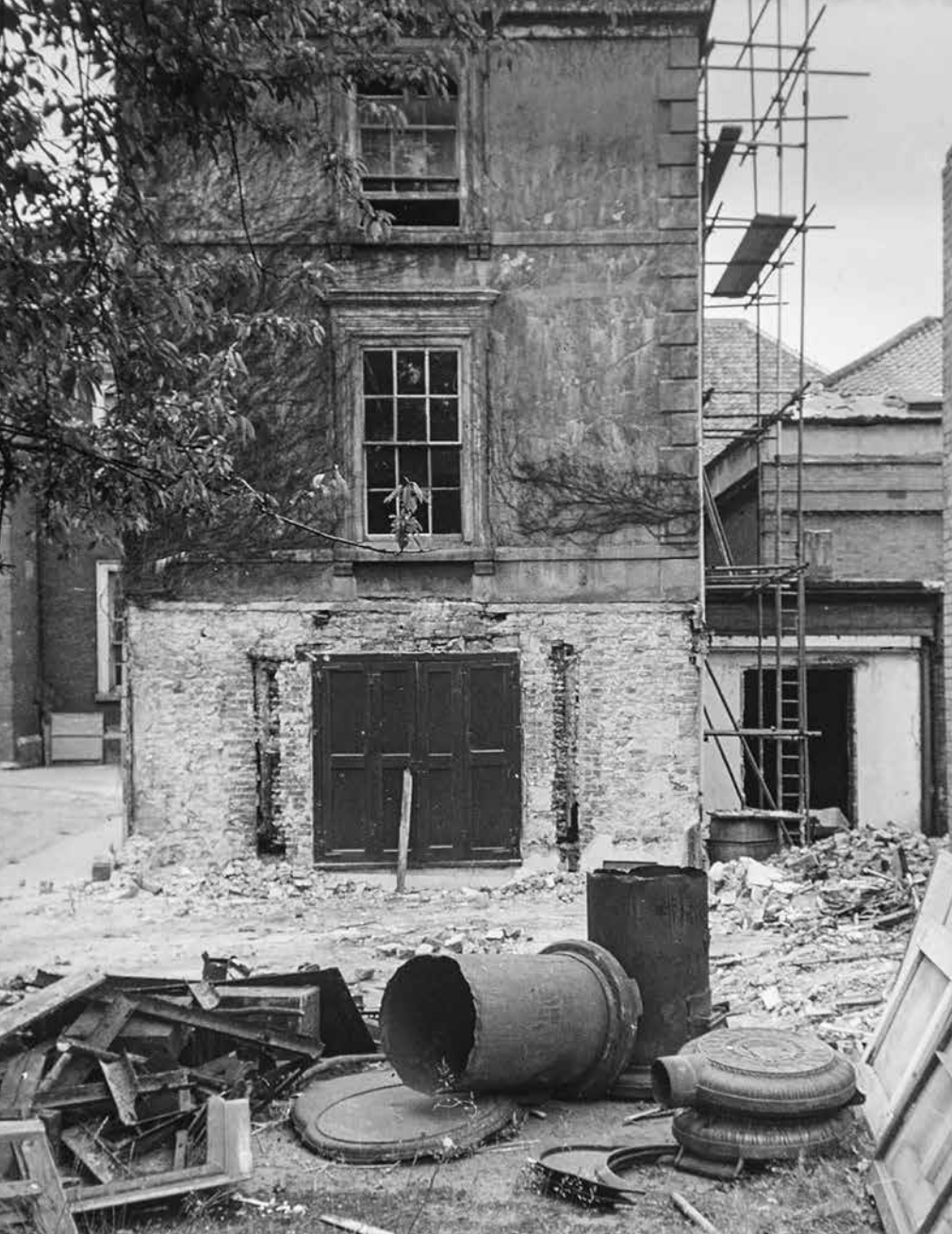
A series of photographs from 1949 recording the renovation work done to the Assembly House when various elements of the older buildings were uncovered. These included wall cores believed to be from Hobart's original Chapply Field House and the remains of a wooden, 12-light Tudor window buried behind a screed coating in the north wall of the west wing.
