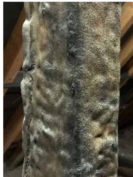
Surviving original oak timbers, so sound and fire-hardened they were retained in the roof structure.
